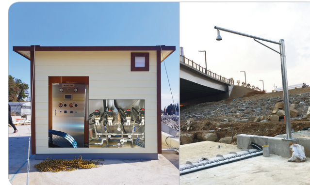
5. Supersonic Water Gauge, Control Chamber Installation
