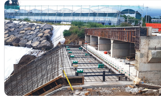
3. Geo Dam Installation
