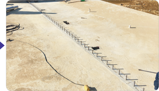
4. Clamping Plate Installation
