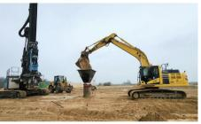
Step 4 Steel casing withdrawn under vibrating & Completion of installation
